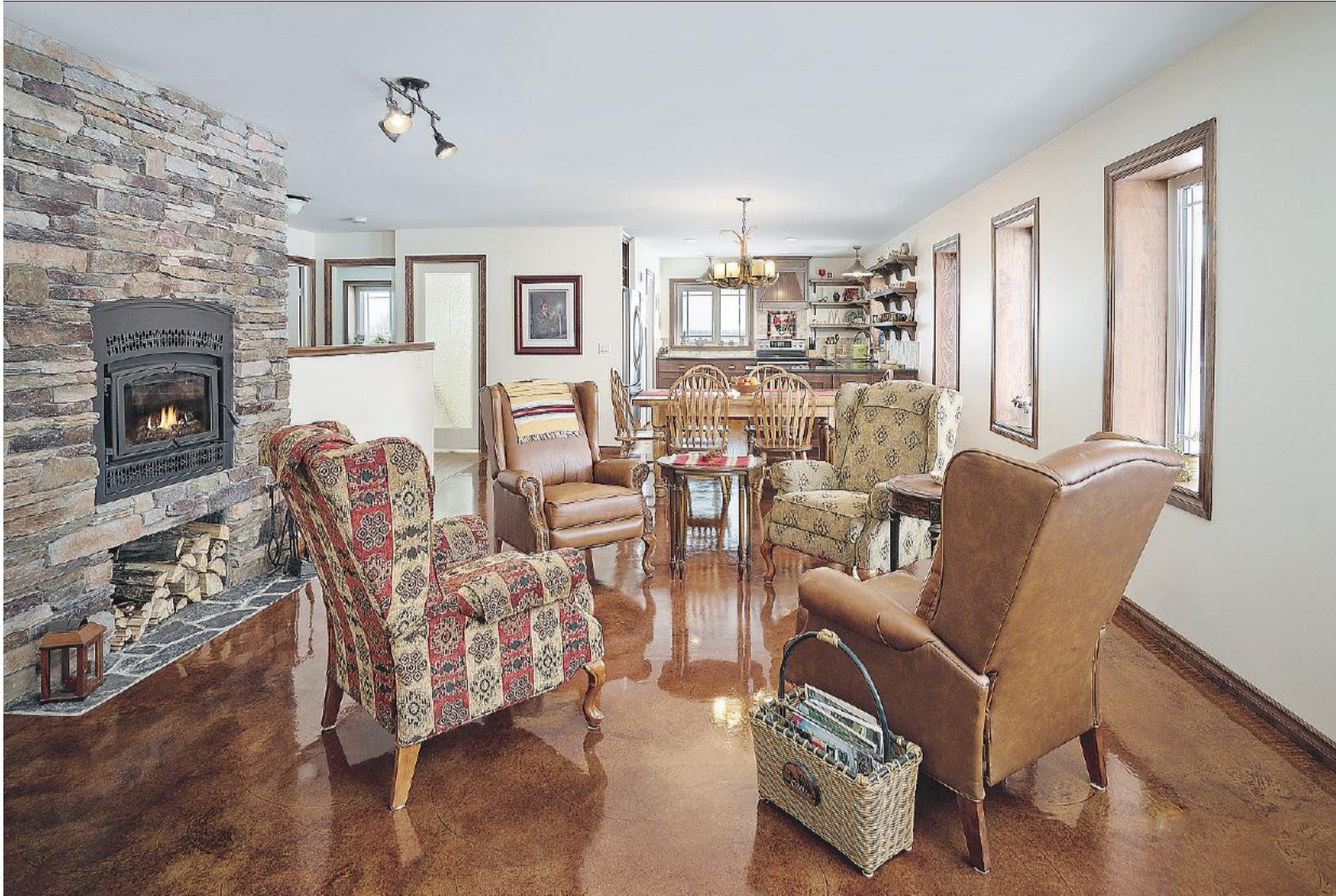
Tim and Lucie Heins' home has a two-inch concrete floor in the dining room/living room area for additional mass heat gain in the front half of house.
