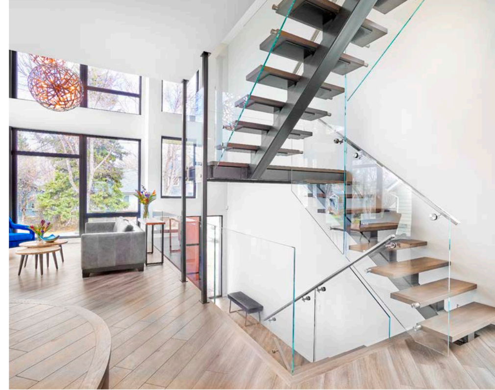
Quarter-sawn, solid oak treads adorn the floating staircase enhanced by 10ml. glass with stainless steel railings and standoffs, providing an airy and elevated ambience.
