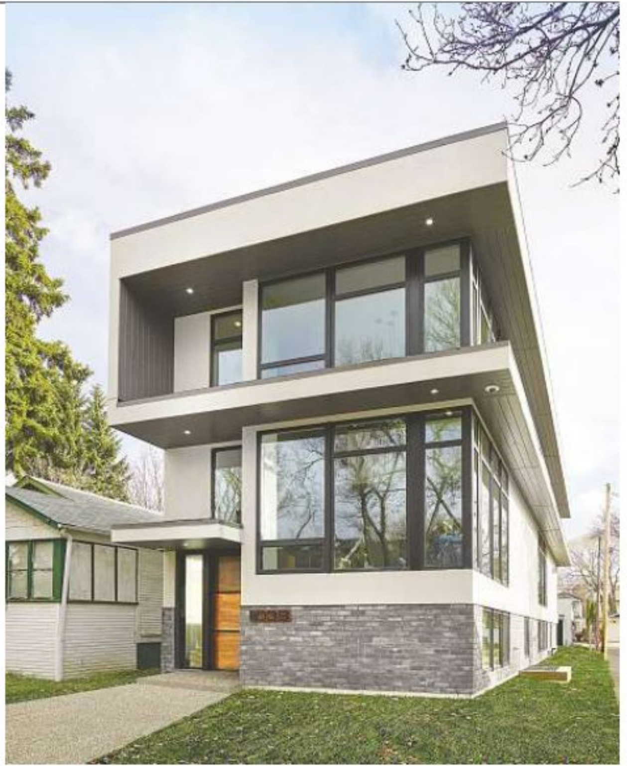
The 4,489-square-foot home in Garneau draws on clean lines and green features. PHOTOS: EFFECT BUILDERS
